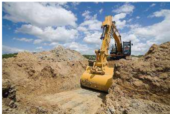
NO. 2 LAYING OF THRUST BED
