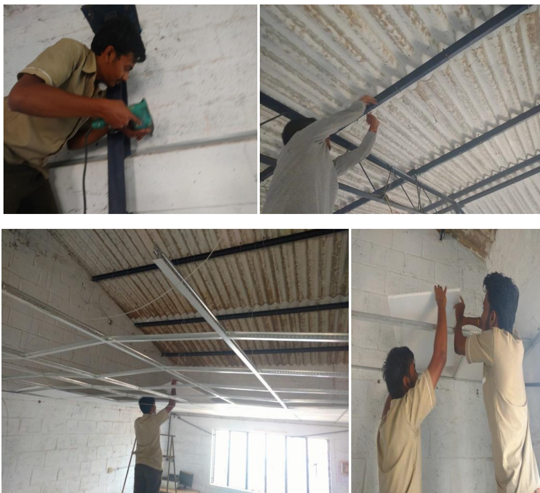
Figure 3: Construction Process - Installation of EPS False Ceiling
