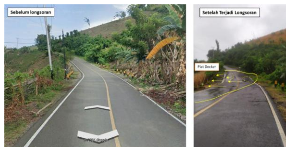
Figure 1: Slope Conditions Before and After Landslide
