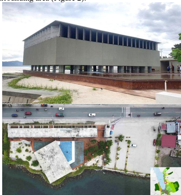
Figure 2: Location and Setting of the Nurul Yaqin Mosque in Palu City Source: Field Data
