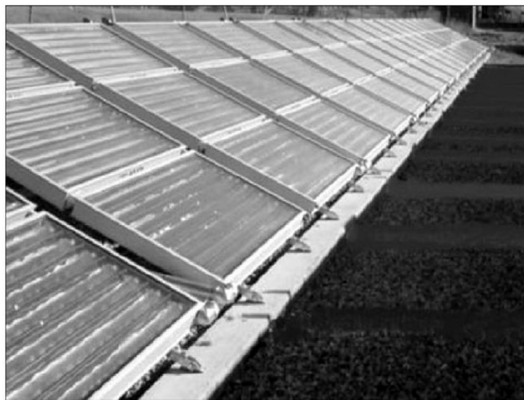
Figure 7: Field installation of CPC panels [4]
