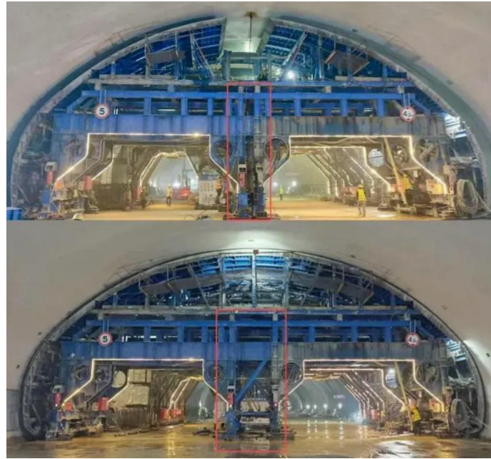
(b) Detailed view of the roof mould and some columns of the large span second liner platform car Figure. 12 Large span second lining trolley site construction plan.
