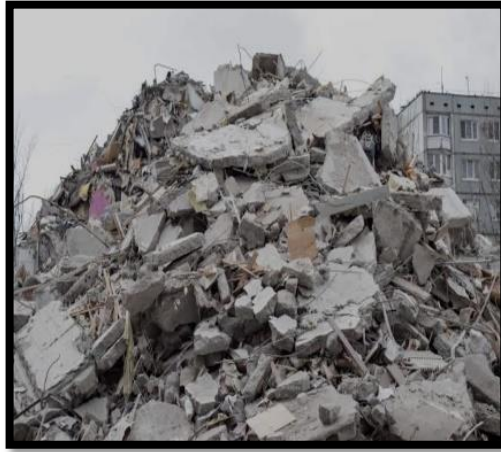
Figure no.02- C and D waste
