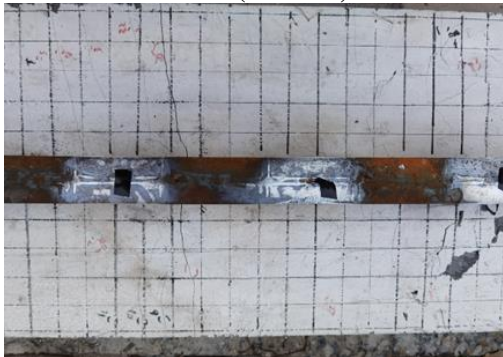
Figure 2.32 Main crack No. 26 (inverted)
