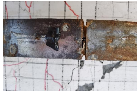
Fig. 3.21 Lower chord fracture
