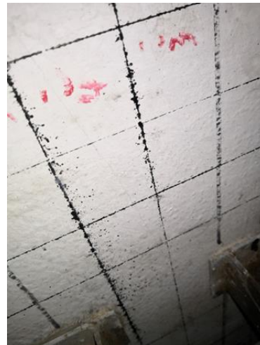
Figure 2.16 Mid-span concrete slab bottom (Grade 7)
