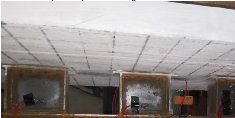
Figure 2.16 Mid-span concrete slab bottom (Grade 7)
