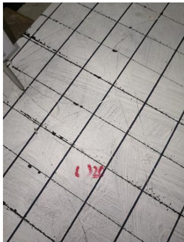
Figure 2.16 Mid-span concrete slab bottom (Grade 7)
