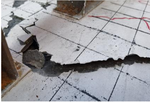
Figure 2.30 Peeling place of the left bending shear section of the bottom of the concrete slab (inverted)
