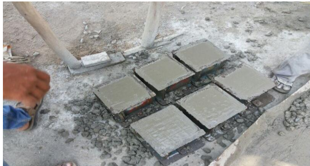
Slump Test of concrete
