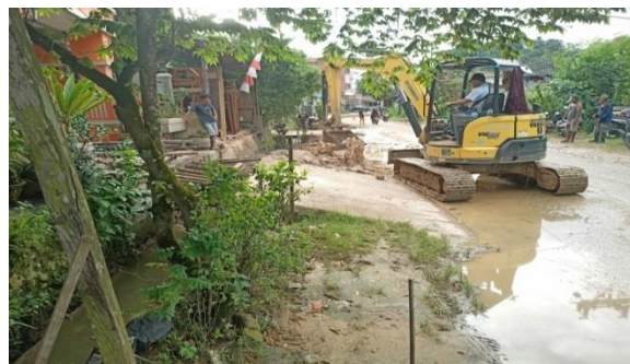
Figure 2. Excavation of Drainage Channels.
