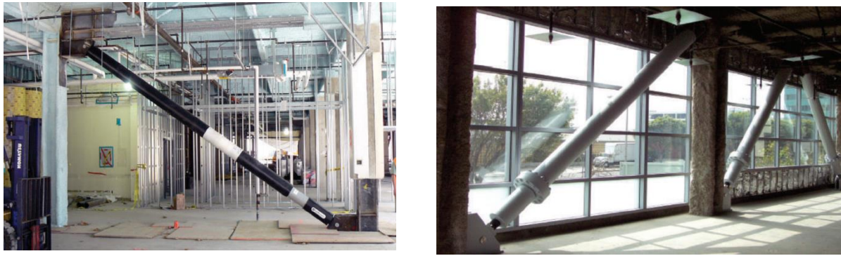
Figure 1: Viscous damper
