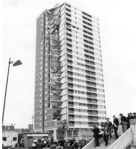
Figure1.1: Ronan Point building after 16 May 1968 collapse
