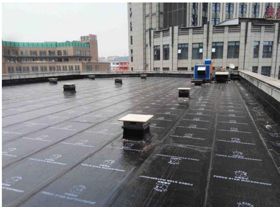
Figure2: Roof waterproof construction
