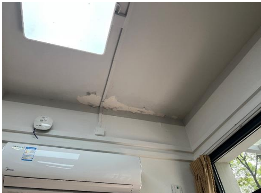
Figure1: Roof leakage
