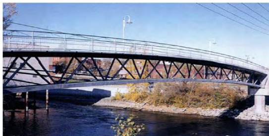
Fig 7: Canada Sherbrooke Overpass
