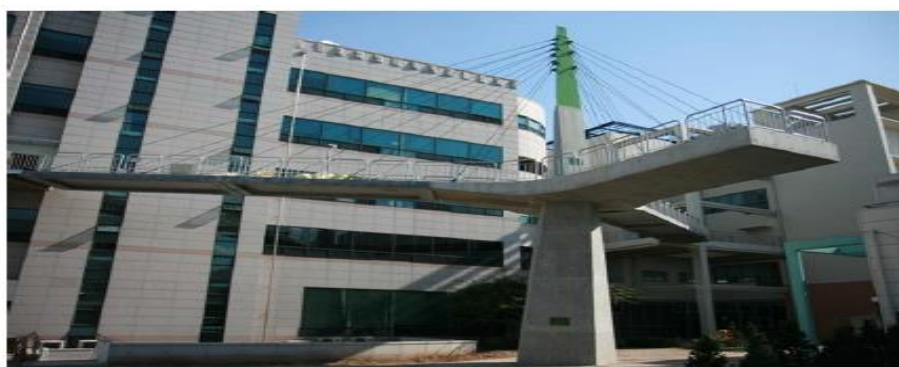
Fig:6 World's first cable-stayed UHPC pedestrian bridge, constructed in 2009
