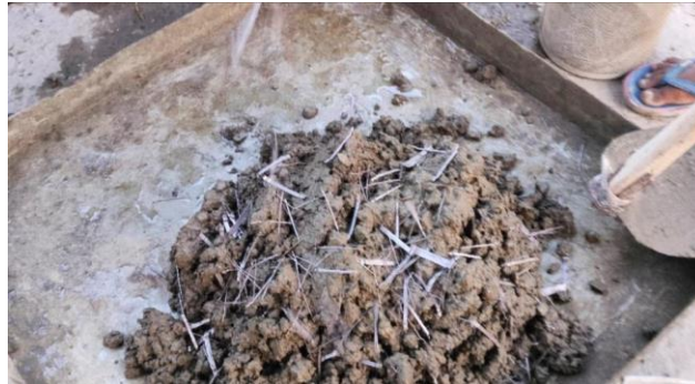
Fig. Preparation of Reinforcement Mesh
