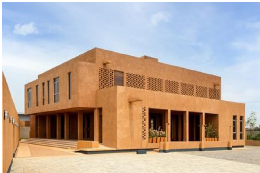
Figure 2: External view of Abijo Mosque, Lagos, Nigeria Source: Abijo mosque / Patrickwaheed design consultancy, 2021
