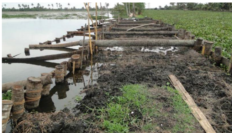
Figure 4. Bund Construction in Kuttanad
