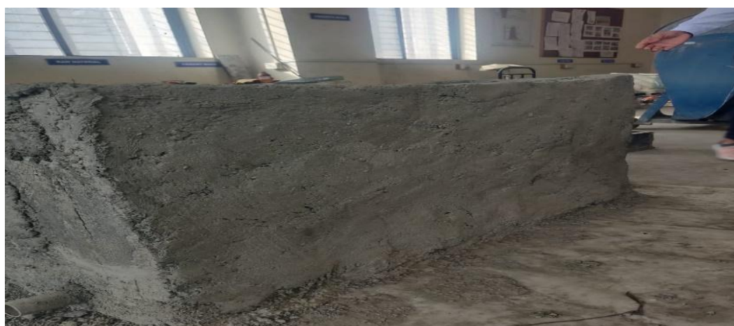
Fig. Showing details of completed tank
