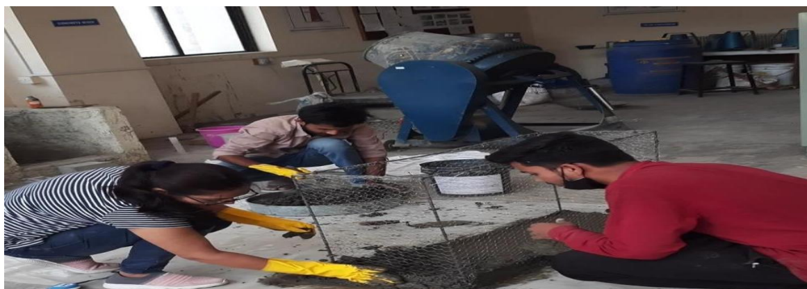
Fig. Showing details of applying mortar
