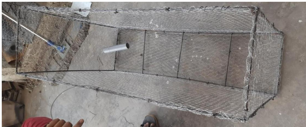
Fig. Showing details of Grid of bars & chicken mesh
