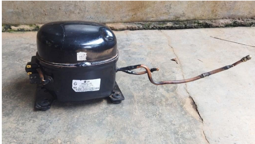
Figure 2: Compressor
