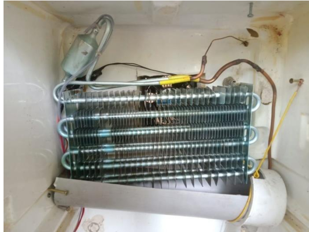
Figure 4: Finned type evaporator
