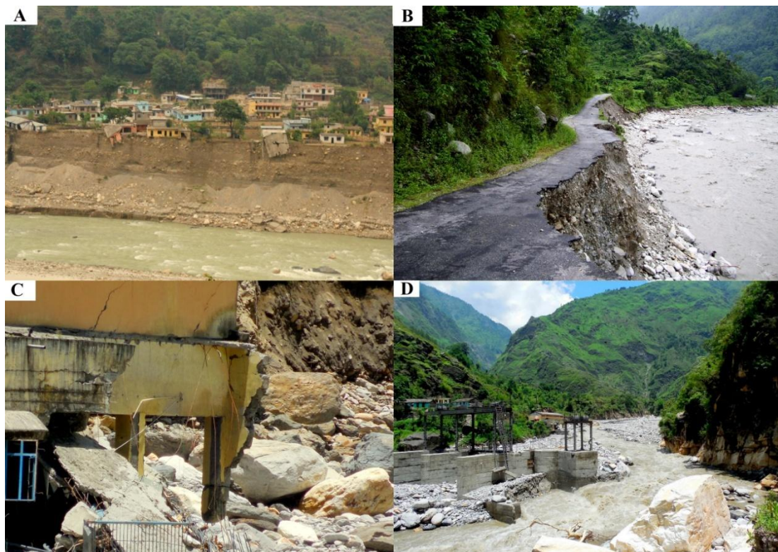
Plate-2: Impact of flash flood and mass wasting disasters in district Pithoragarh: (A) at Ghatta Bagar (2013), (B) at Mori village (2013), (C) at Dani Bagar (2016) and (D) Himalaya Hydro Power Project Dam damaged at Bali Bagar (2018) (based on field survey).
