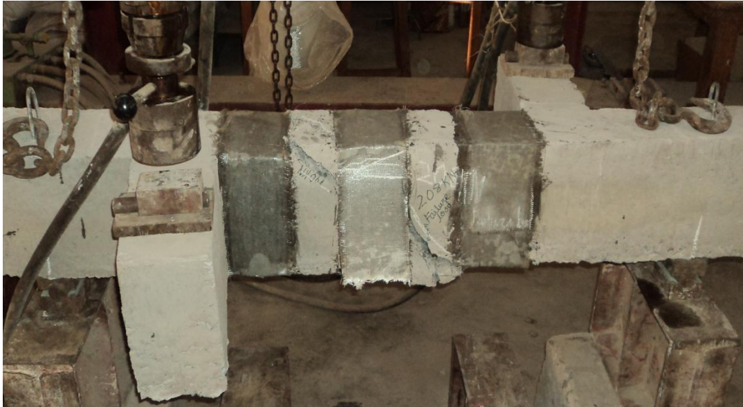
Figure 13 shows the failure of the retrofitted beam, when the GFRP sheet was still intact.
