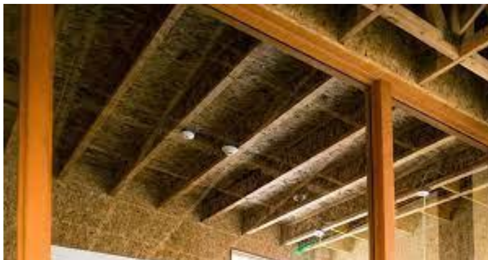
Figure2: Wood I-Joists for Ceiling
