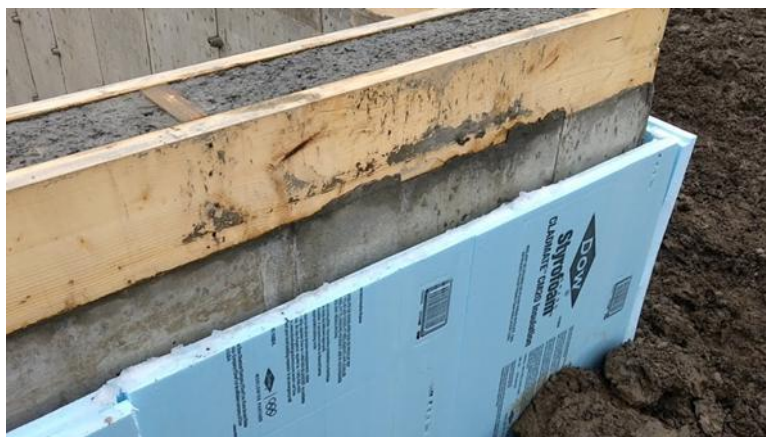
Figure1: Insulation for foundation before backfilling
