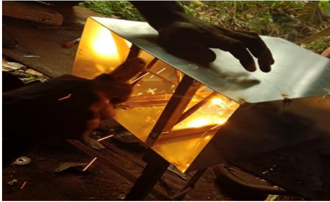
Fig.5.Fixing the connector by drilling
