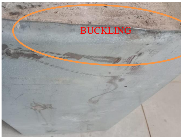
Fig.9 Buckling formed in the wall
