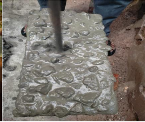
Fig.6 concrete placing & compaction
