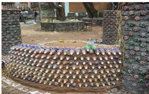
fig 7. Laying Plastic Bottleswithrope
