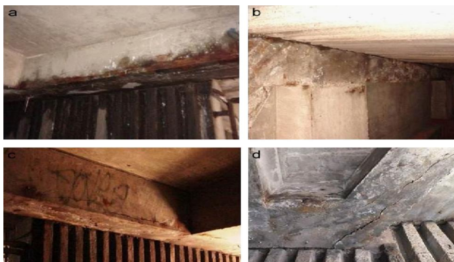
Figure 1: Concrete deterioration between spans (a) seepage, (b) efflorescence, (c) concrete cover delamination, (d) wide cracks[2]
