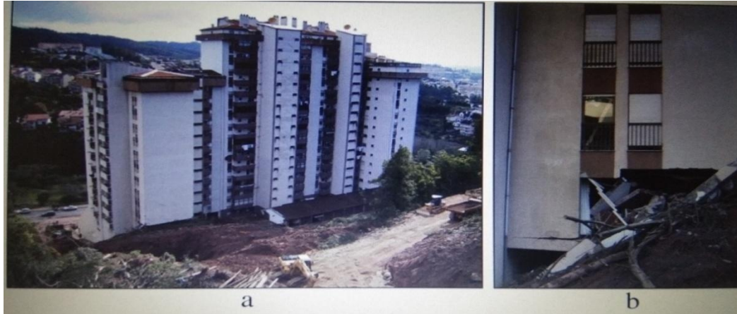
Fig. (a) Rear (West) façade of the building, a few days after the accident. (b) Detail of the total collapse of the outer columns of the damaged rear body of the building.
