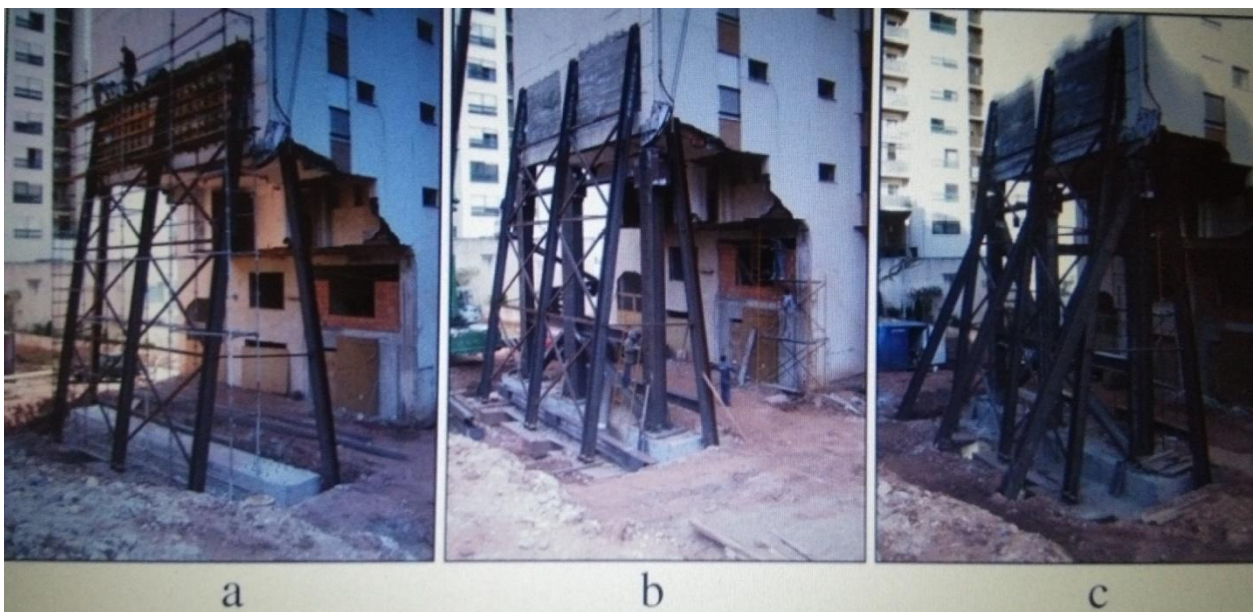
Fig. (a) Foundation for the retrofitting steel frame and shear wall. (b) Assembling the retrofitting steel frame. (c) Additional bracing steel shores
