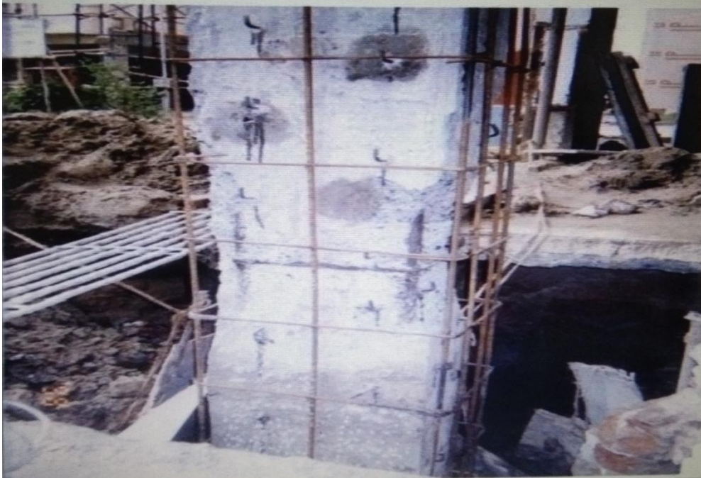
Fig. Jacketing of columns from the footing level.
