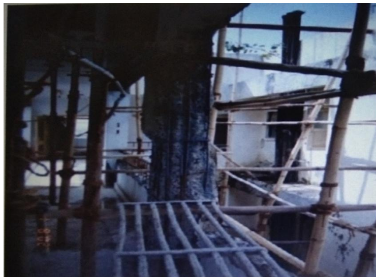
Fig. Column rebars with anti -corrosive coating
