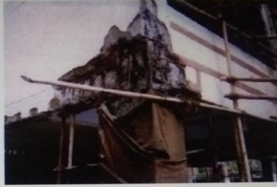
Fig.1 De-lamination of beam concrete cover due to rebar corrosion. Fig.2- Severe corrosion and spalling of beam - column junction due to poor workmanship and in-adequate cover at GF level.
