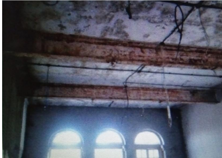
Fig. Roof Leakages
