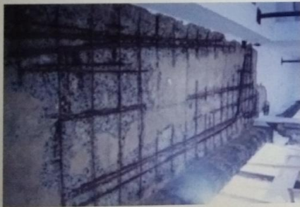
Fig.3 De-lamination of concrete cover due to severe corrosion of rebars of roof slab. Fig. 4- Continuous wide crack in column due to corrosion of longitudinal steel at concrete cover depth.
