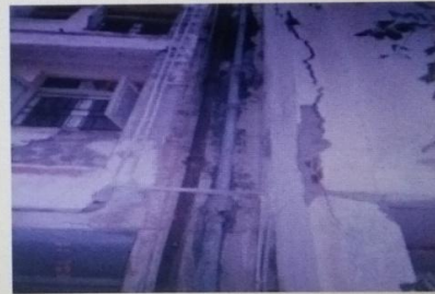
Fig.3 De-lamination of concrete cover due to severe corrosion of rebars of roof slab. Fig. 4- Continuous wide crack in column due to corrosion of longitudinal steel at concrete cover depth.
