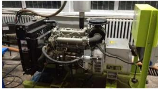
Figure1: Diesel Engine Generator Where Experiments Are Conducted
