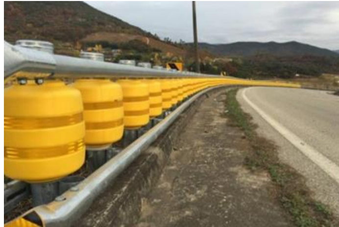
Figure: 1 Rolling Barriers on horizontal curve
