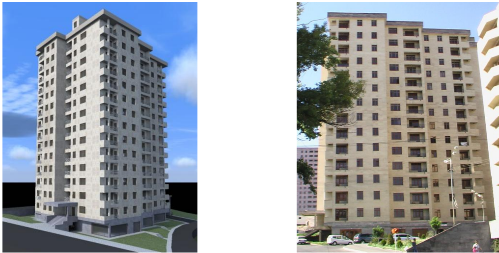
Figure 9. Design view of the 15-story base isolated apartment building of residential complex “Avan” and its current view
