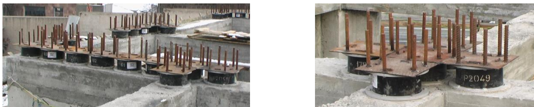
Figure 10. Examples on installation of rubber bearings' clusters in the 15-story base isolated apartment building “Avan”
