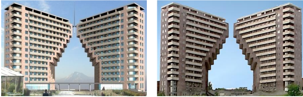
Figure 6. Architectural design view of the 18-story base isolated buildings of residential complex “Northern Ray” from the Northern side and its current view from the Southern side
