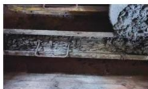
Fig-6 FILLING THE CONCRETE
