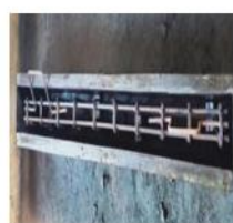
Fig-5 Placing Reinforcement
