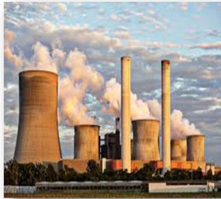
Figure 1. Industrial RC chimney
