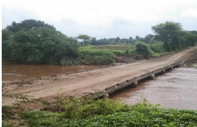
Fig. 3 Naved-Darapur River Bridge
