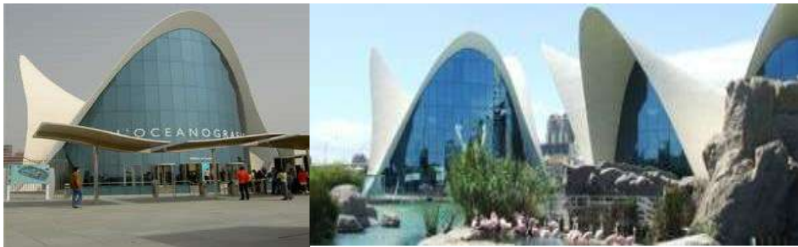
Fig. 2: SFRC shells made in the European Oceanographic Park in Valencia [2]
