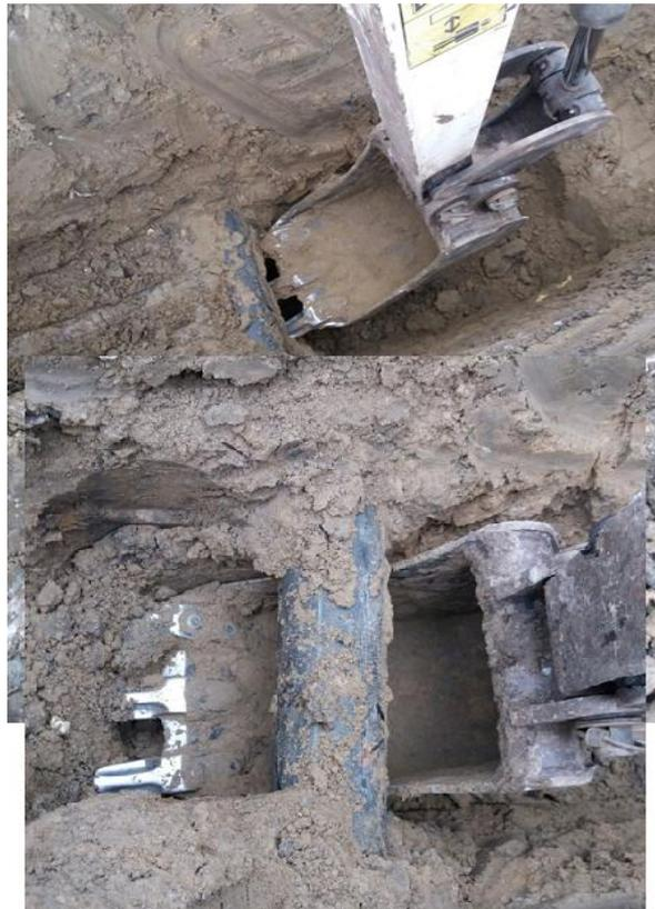
**Fig.11.** Actual situation of accidentally applying stress on the PE 100 polyethylene pipe by the excavator bucket
