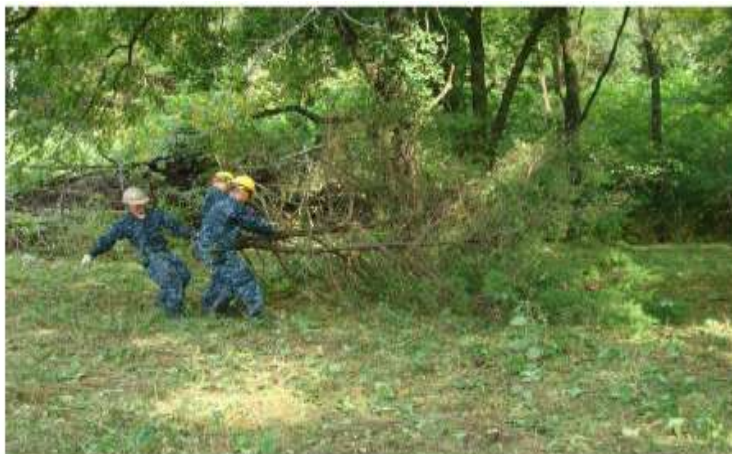
Figure 3: United States Navy Seabees Clearing the Site
